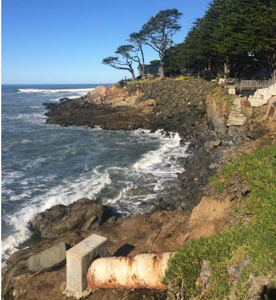
Residential Structures in Tsunami Risk Area
