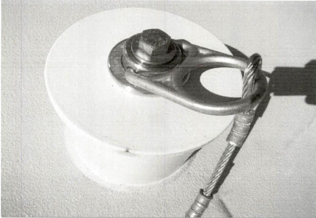
This view shows one of the two fall protection cable anchors with a small rust point.
