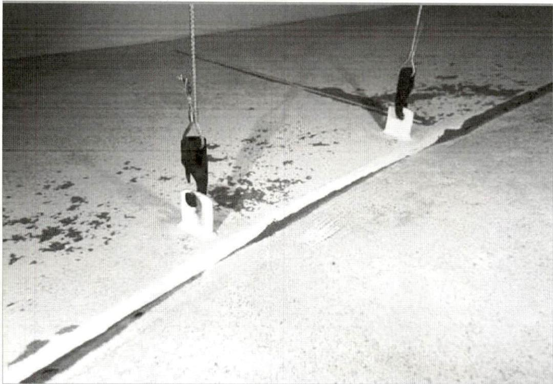
Level gage guide wires and attachment tabs on the interior bottom.
