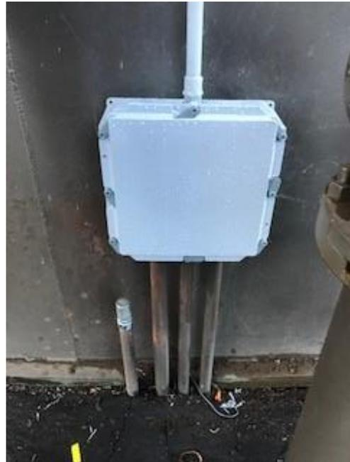
*Figure 3 Rusted electrical pull box*
