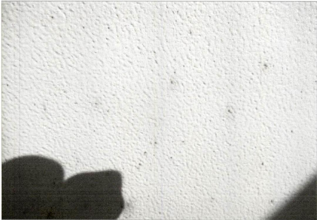
This close view of the mid shell at the exterior ladder shows some scattered corrosion found where holidays are present in poorly wetted coating.
