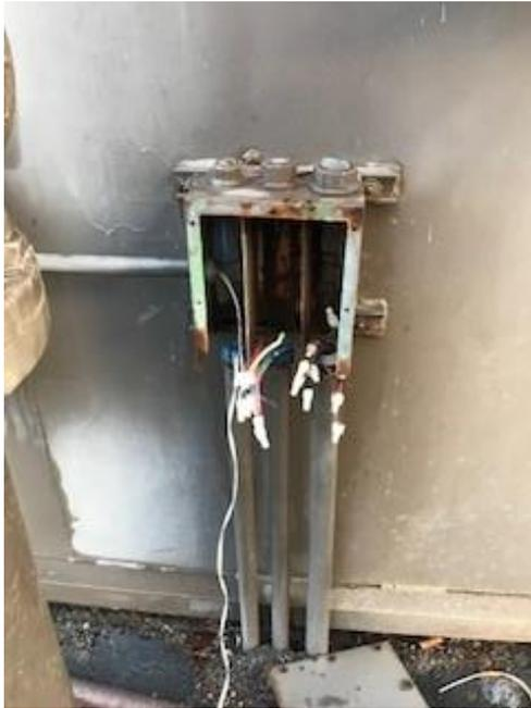
*Figure 2 New electrical pull box*
