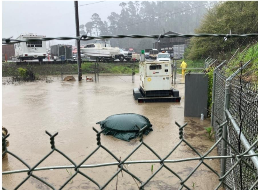
Figure 7 This was the last photo taken of lift station B-1 during the rains, this was at approximately 8:45. At 9:11 we received the last communication. We were all landlocked at the WWTP shortly after.
