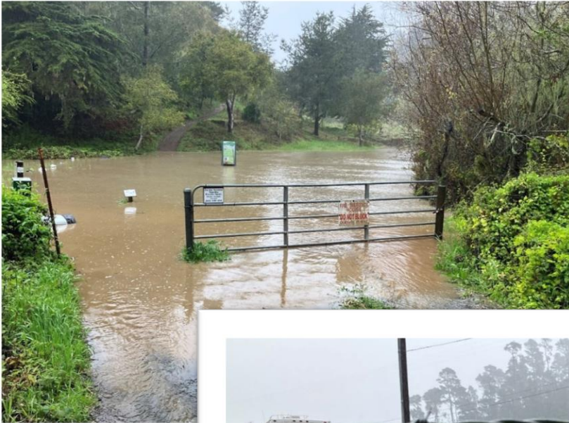
Figure 6 Access road to lift station B during the 3-10 storm.
