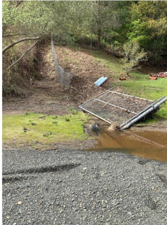
Figure 10 Lift station B new section of fence.
