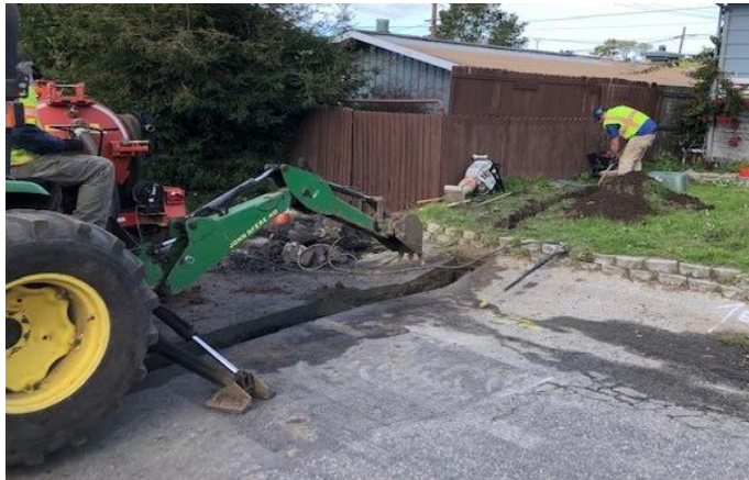
Figure 3 Trenching for new 1" line installation
