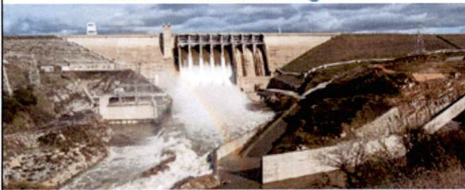
Folsom Dam project funded by Prop 18 - with five spill gates open, releasing water to the American River in Folsom, CA - December 2018
