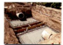
Ivanhoe Irrigation Dist. 69 Main Project
