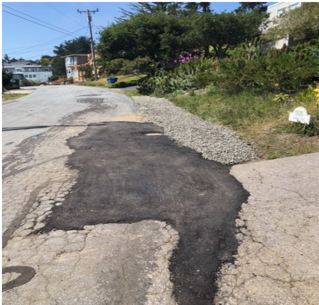
Figure 4 Emmons St after repair.
