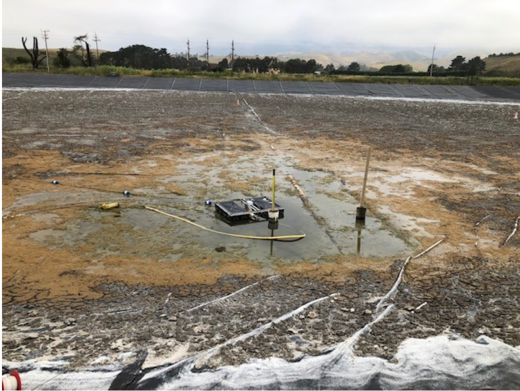
Figure 5 Impoundment Basin nearing completion of closure plan.
