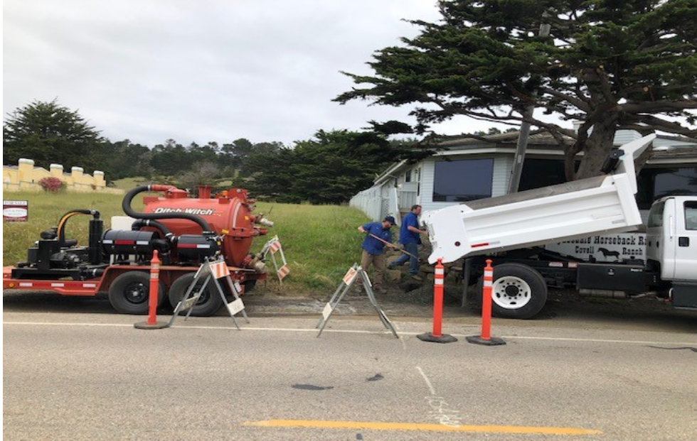
Figure 1 Staff fills road base in after leak repair on MBD.
