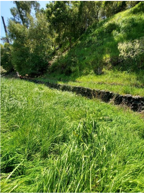
Rock wall; property line (section 8)?
