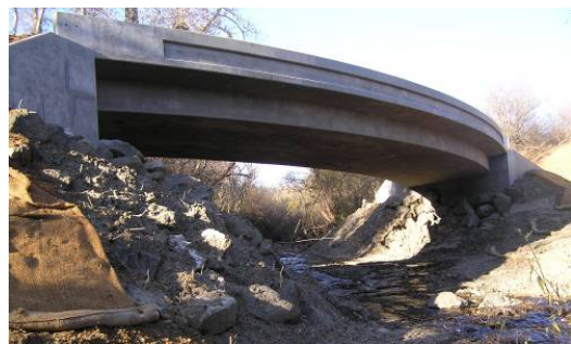
Ferrasci Road crossing before (above) and after (below) replacement
