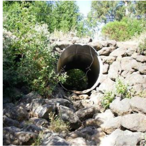
Culvert on Curti Creek
