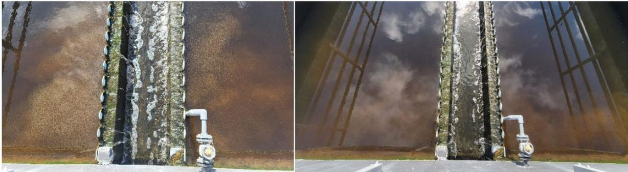
Figure A- Clarifier before (left) and after (right) polymer additive
