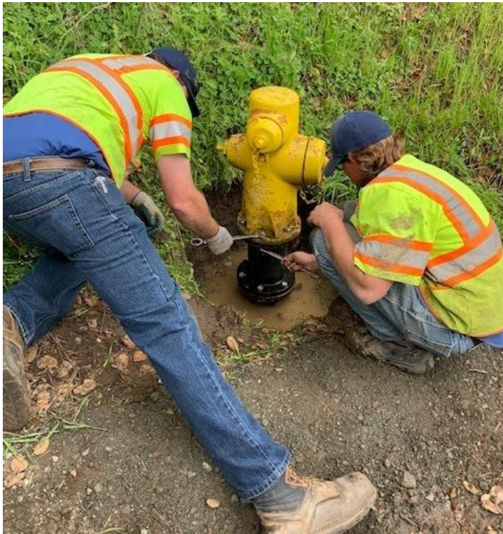
Figure D - Repair to a leaking fire hydrant
