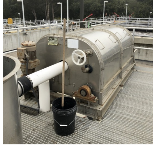
Figure 11: Sludge thickener
