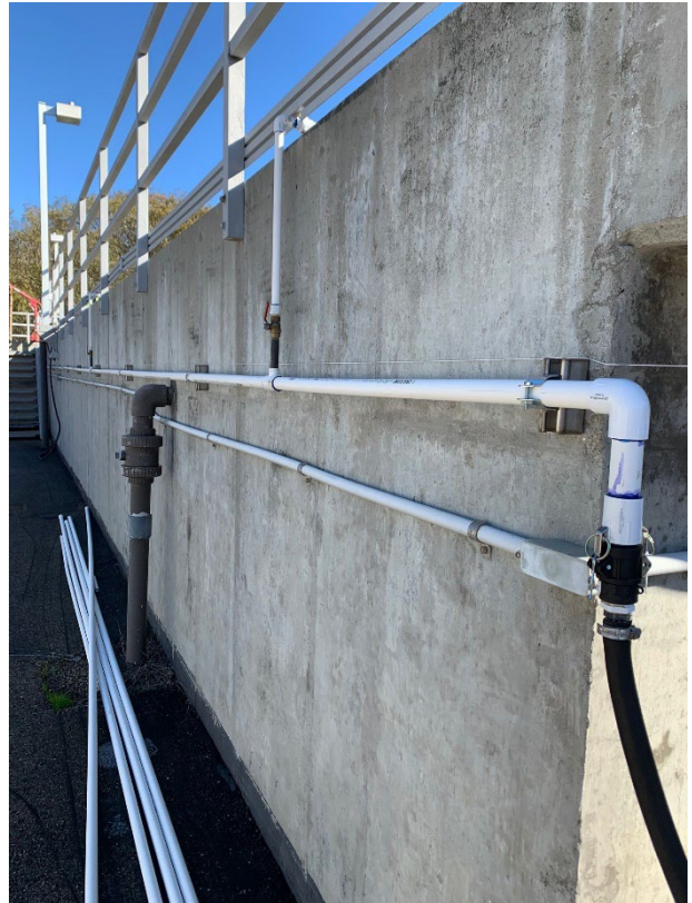
Figure A - New polymer piping
