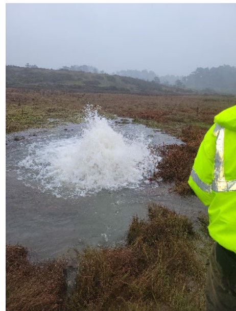
Figure E San Simeon Transmission Main Break
