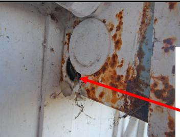
Unprotected / unused opening(s) through the SIDE of the MAIN ELECTRICAL PANEL needing to be sealed for safety per standards. This will help prevent critter intrusion into the electrical panel.
