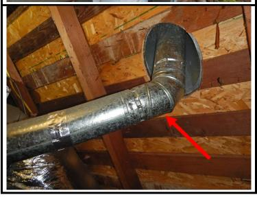
Missing the proper strapping at the furnace vent piping in the attic at the horizontal to vertical transition through the roof
