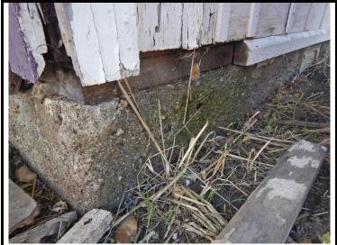
Some deterioration / spalling of the original concrete foundation. This appears typical of the age. However, upgrades are recommended to help prevent additional deterioration, damage or compromise of the concrete.
