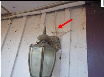
Improper wiring / Exposed electrical wiring or "Romex" found not installed to minimum standards subject to physical damage not in a conduit or raceway per standards. Safety Hazard: ON THE EXTERIOR AT THE FRONT ENTRY LIGHT
