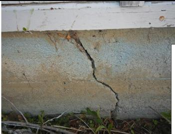
Some moderate cracks and/or displacement of the raised concrete foundation perimeter stem wall noted in multiple areas. This may be indicative of unusual settling or movement of the soil around the foundation.
