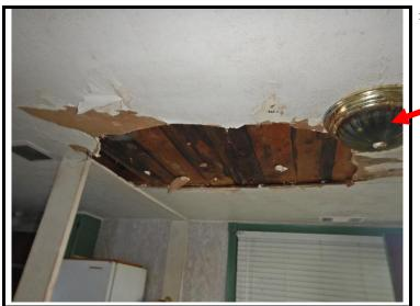
Heavy active water leaking and damage found in areas of the interior ceilings / wet today.
