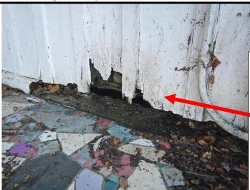
Areas of excessive moisture and / or bug type damage and deterioration found at areas of the structural wood framing.
