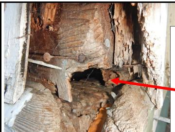
Areas of excessive moisture and / or bug type damage and deterioration found at areas of the structural wood framing.
