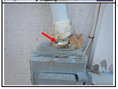
A broken electrical conduit found at an added exterior outlet. Safety Hazard.
