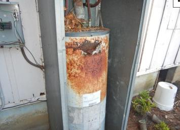
The Water heater is defective, damaged, improperly installed and unsafe.
