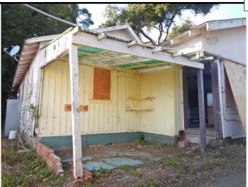
Some moisture damage and defective construction found at the WOOD PATIO COVER WITH FIBERGLASS CORRUGATED ROOF located on the Southeast corner. Recommend removal.
