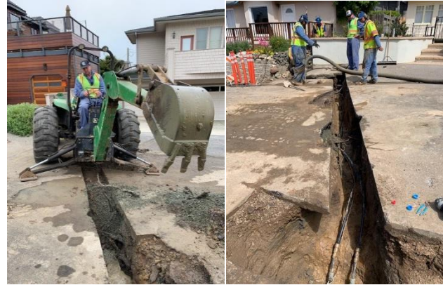
Figure 3 Water Dept staff onsite for a leak repair
