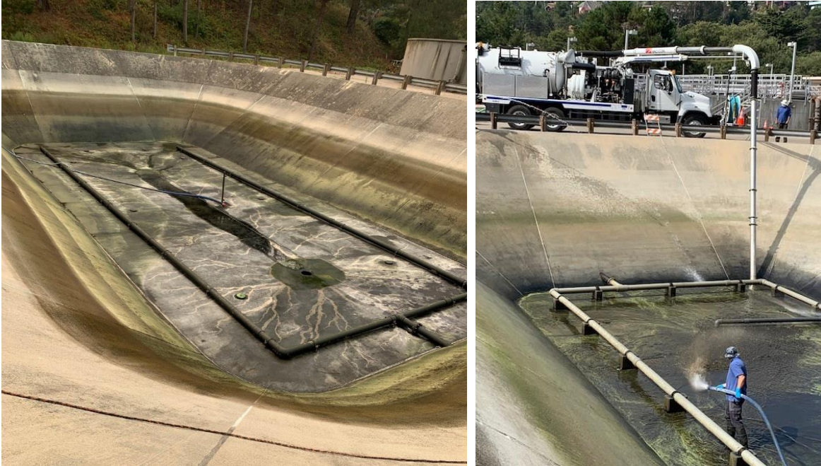
Figure 2 Cleaning out the effluent holding ponds
