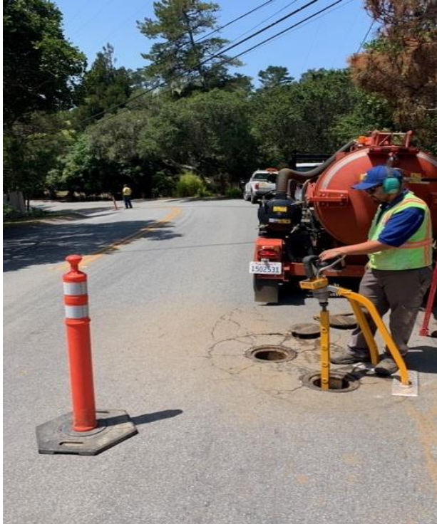
Figure 6 Valve exercising activities
