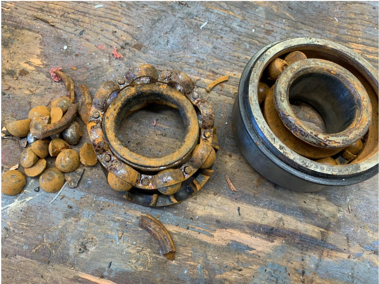
Figure 5 Bearings out of a lift station pump.
