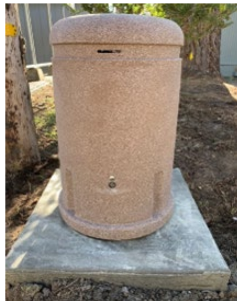
Final assembly of the air-vac enclosure
