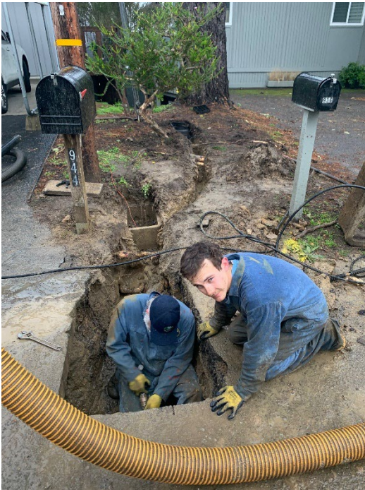
Operator-in-Training, Owen looks on while final installations are being made
