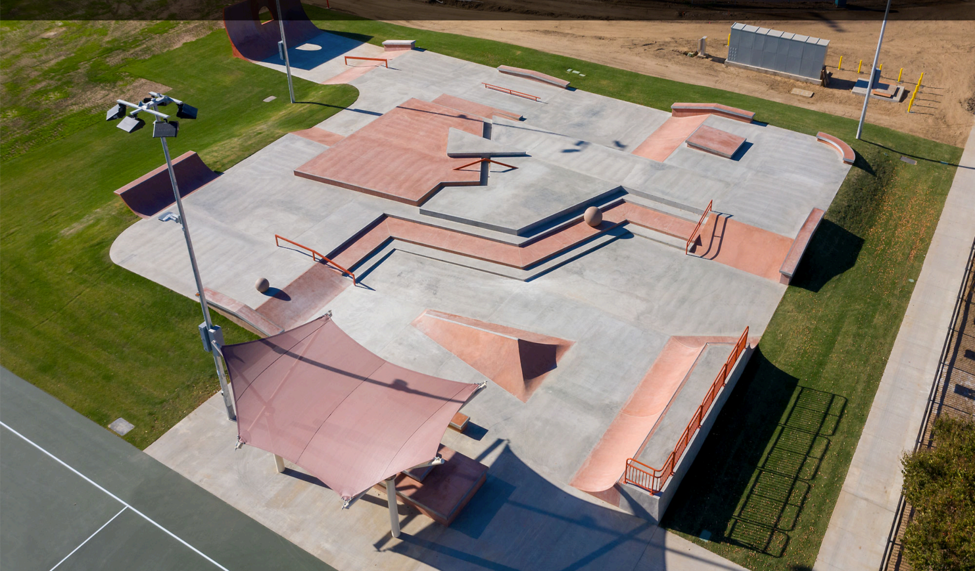
La Puente, CA – Tech street plaza, lighting, shade structure, iconic over-vert wall
