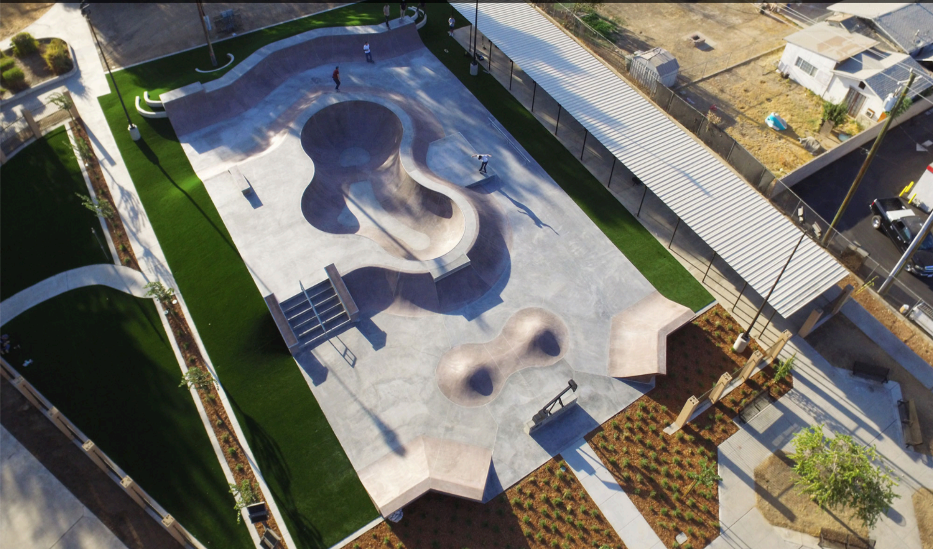
Oildale, CA – Street, flow & bowl, w/colored concrete, synthetic turf & entry sculpture – 40/60
