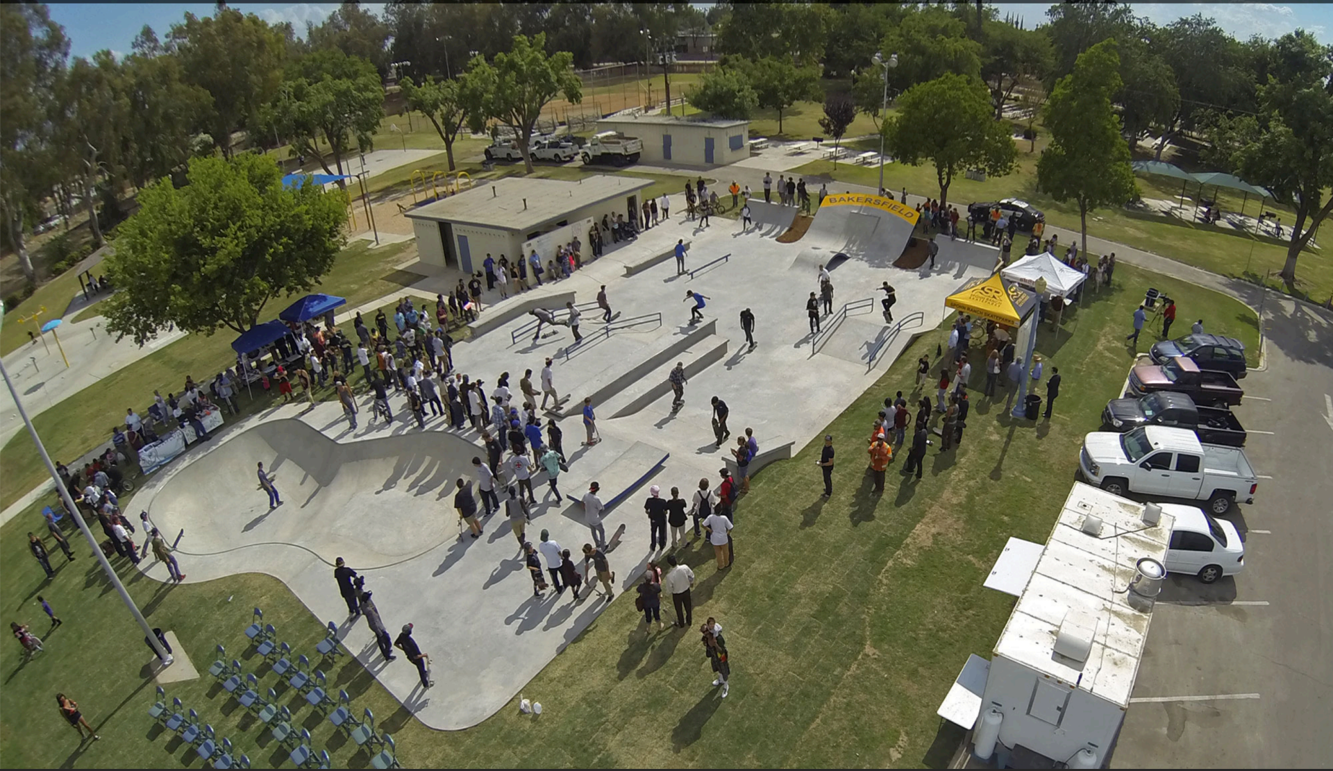
Bakersfield, CA – Street plaza and beginner bowl, lighting & iconic art bank – 70/30 Ratio
