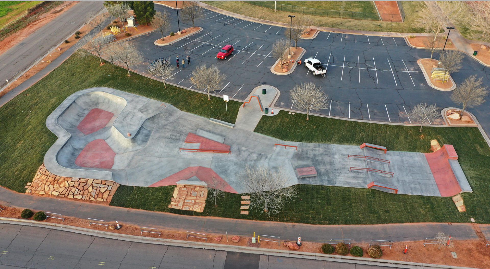
Ivins, UT – Street plaza and bowl, w/colored concrete, rockscape and entry arch – 70/30 Ratio
