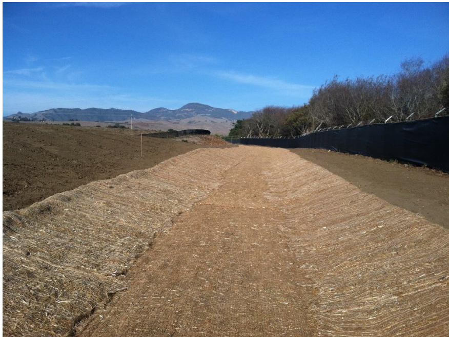
12/1/2017 Lined Swale along East Side of Impoundment Basin
