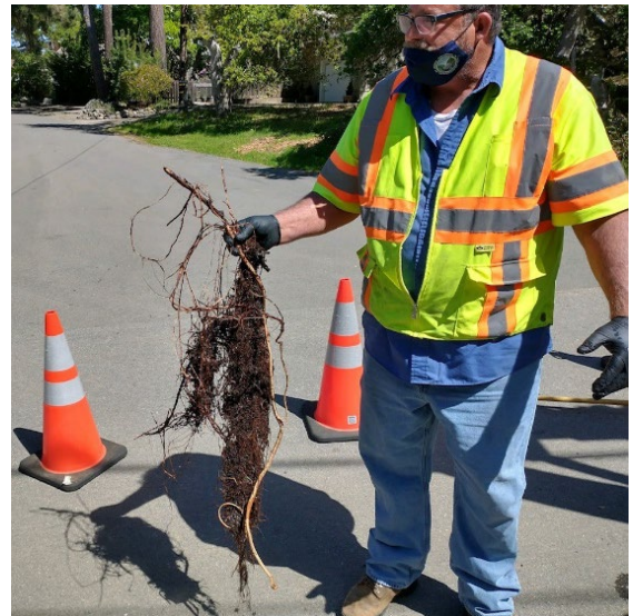
Figure C - Root intrusion pulled from the collection system
