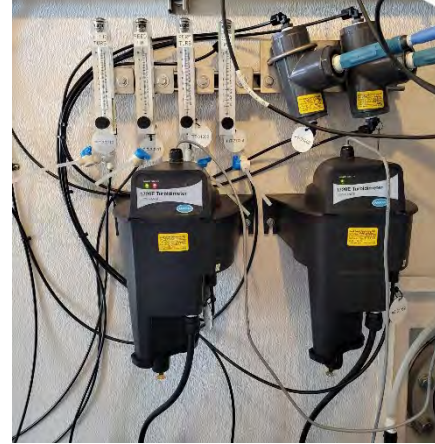
Figure F - Turbidimeters in the micro-filtration train were included in the calibration efforts.
