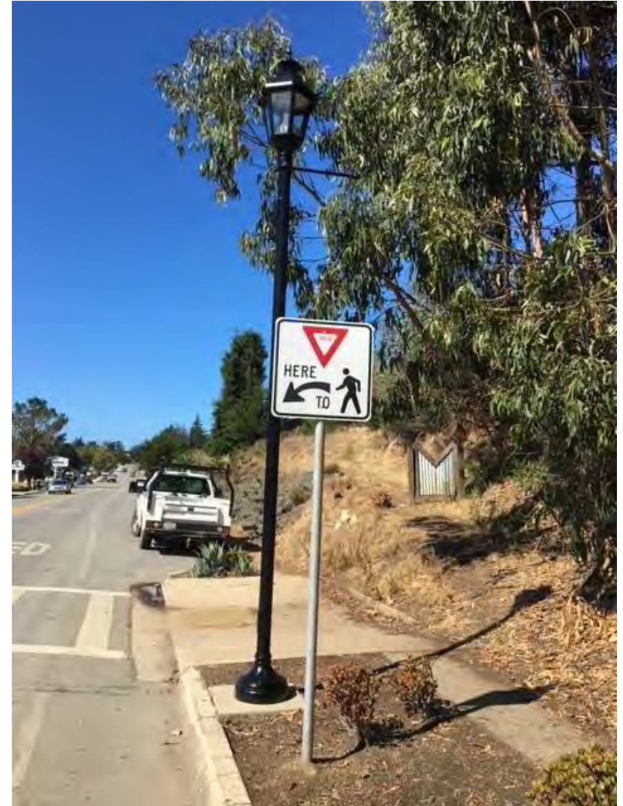
New Light Installed
