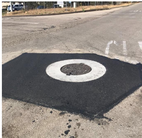
Figure 2 Manhole repair at Main/Windsor
