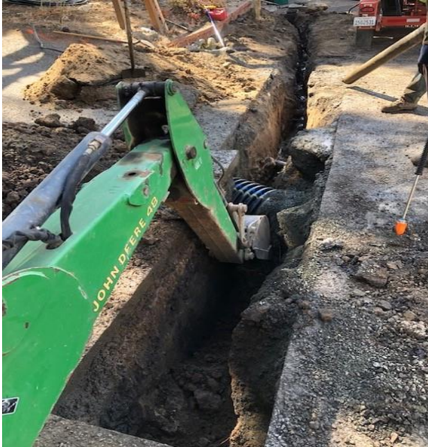
Figure 1 Hillcrest line replacement
