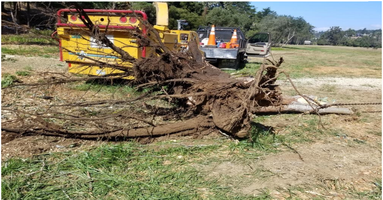
Figure 4 Removed segment of tree during repair
