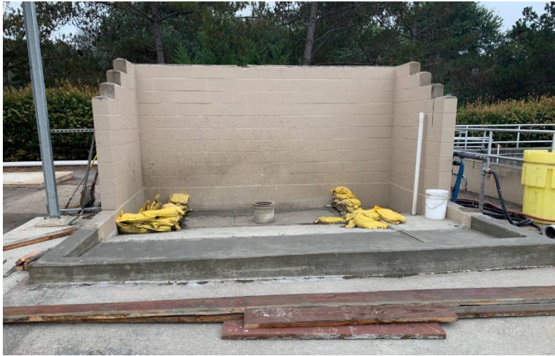
Figure A - Newly installed concrete berm at WWTP dump station
