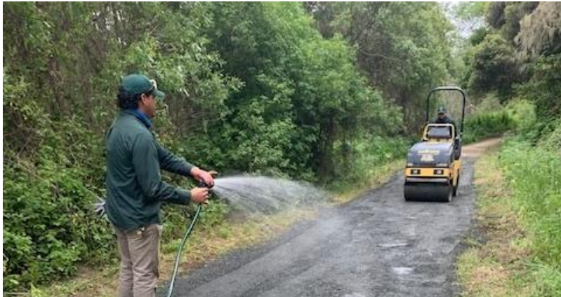
Debris hauled away, base material delivered, laid and compacted
