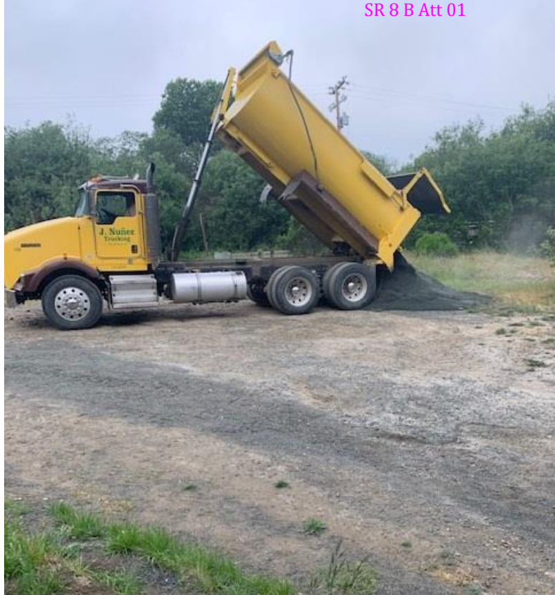
Debris hauled away, base material delivered, laid and compacted
