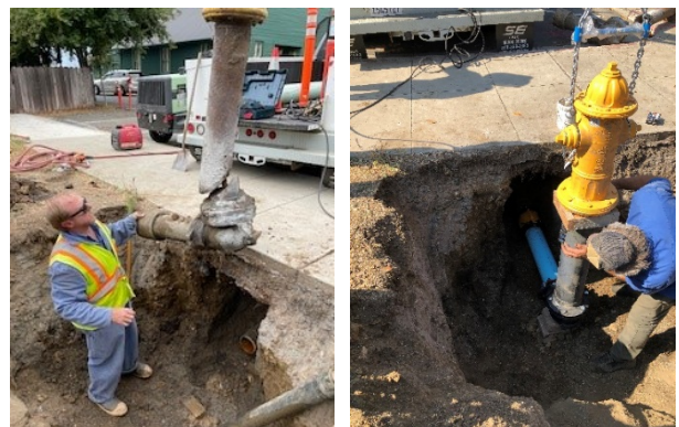
Figure C – Old hydrant removal (left) and new hydrant installation (right)
