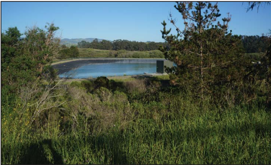
View from Van Gordon Creek Road, looking east at the evaporators and evaporation pond.
