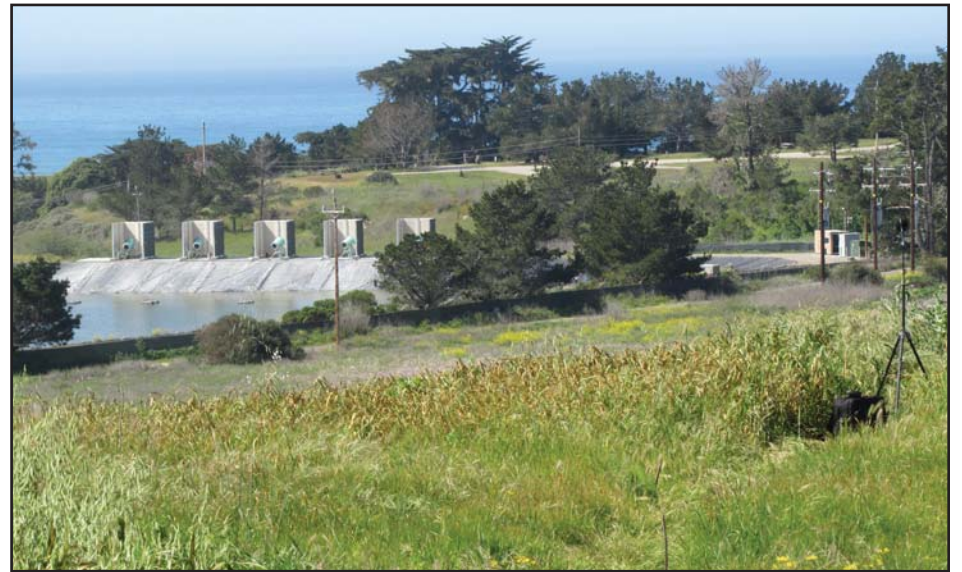
View from San Simeon Creek Road looking south at the evaporators and evaporation pond.
