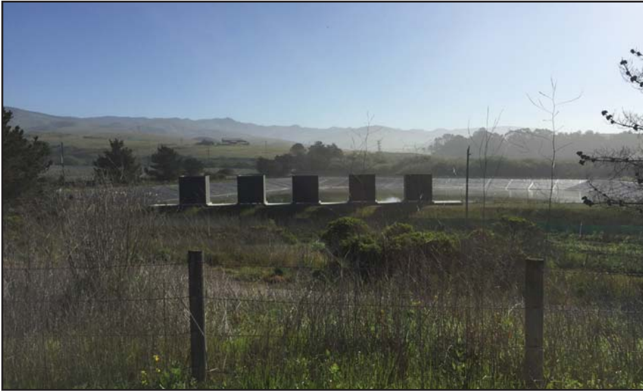
View from Van Gordon Creek Road, looking east at the evaporators and evaporation pond.
