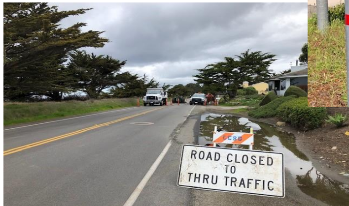
Figure 4 Line replacement underway on MBD
