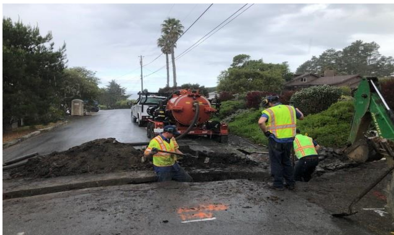
Figure 2 Full line replacement on a wet Warren Street
