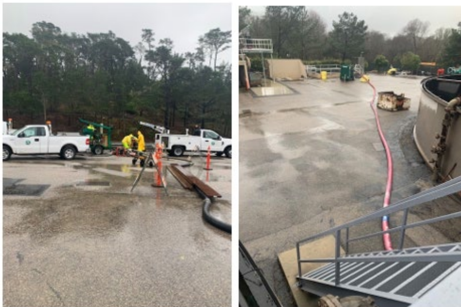
Figure C Staff had to get creative with where excess water was stored during and after the storm
