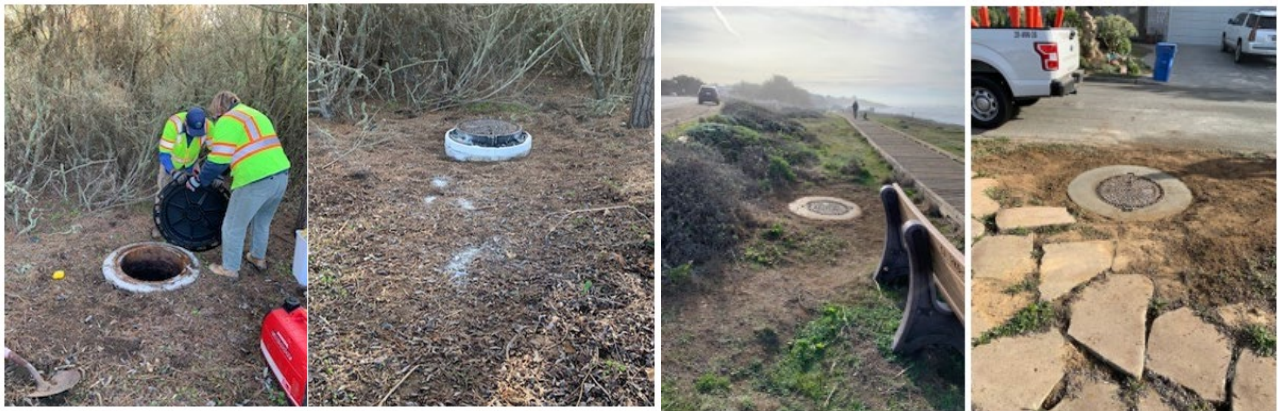
Figure A - New manhole lids and bases
