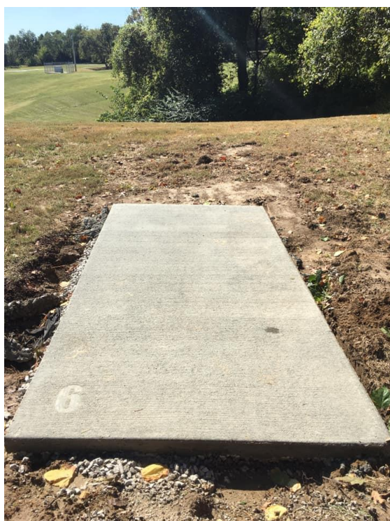
Concrete tee pad, unfinished. One of several tee pad material options.
