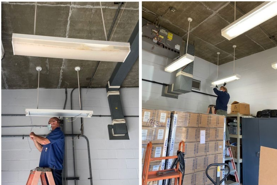
Figure A Replacing lights at the WWTP
