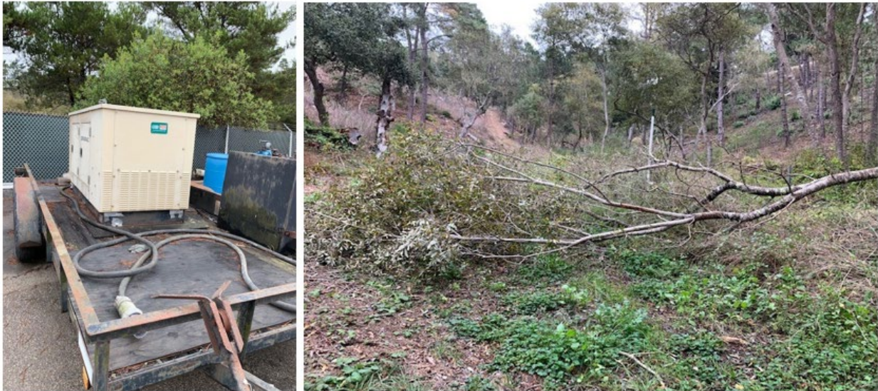
Figure B Old generator (left) and fallen tree (right)
