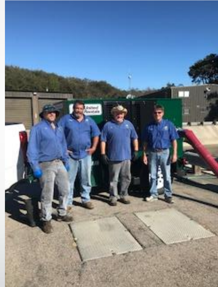
The department installed and tested the new 6 inch pump.
