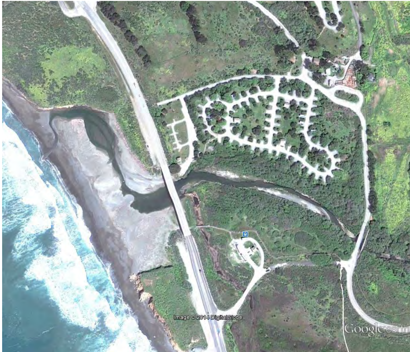
Figure 2 – March 2010 Aerial Photo Showing Discharge to Ocean
