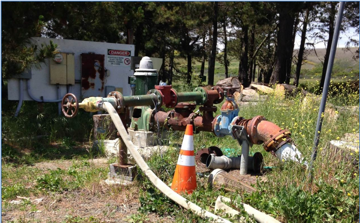
Figure 2-1 Existing Well 9P7
