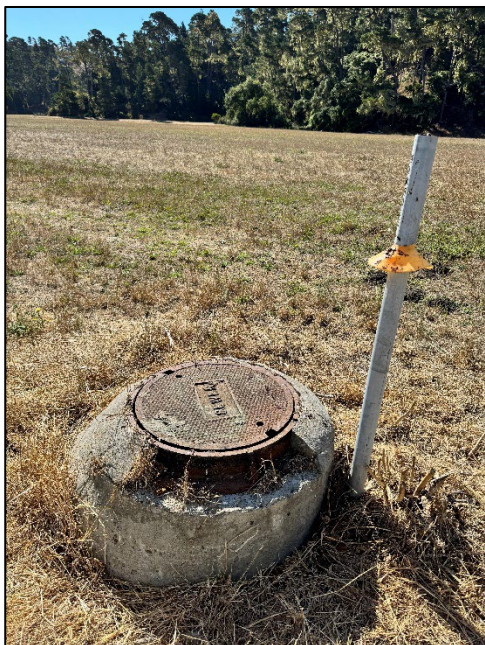
Figure 14: Damaged manhole #1
