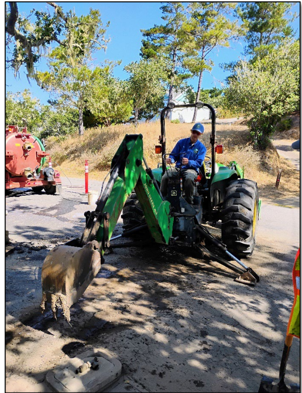
Figure 20: Main Street Repair and Replacement
