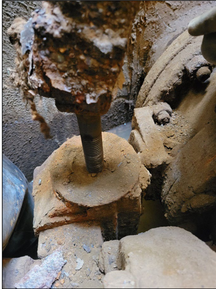
Figure 2: Operator Stem Assembly Close Up
