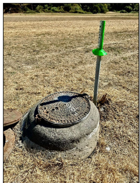
Figure 15: Manhole with new Pamrex lid
