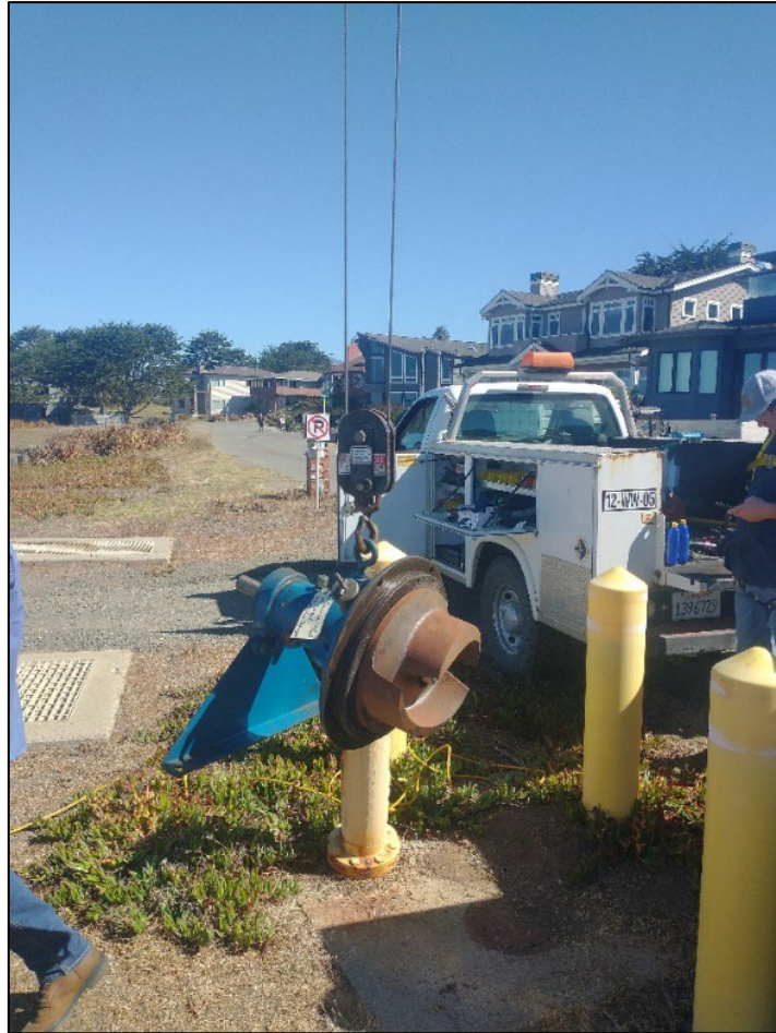
Figure 10: Maintenance at Lift Station A
