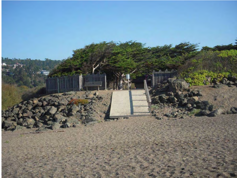
Photo 5: Photo taken from the beach looking landward at the Shamel Park emergency vehicle access ramp. Santa Rosa Creek is to the left.
