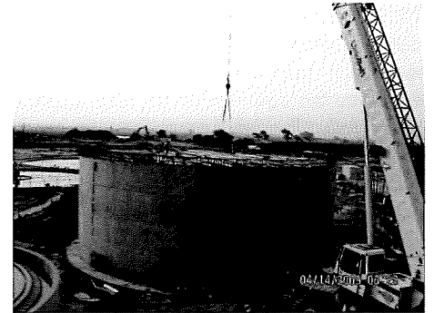
Santa Maria Digester No. 4 Wall and Roof Scaffolding
