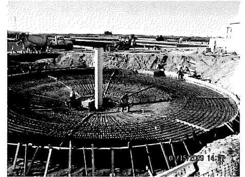
Santa Maria Digester No. 4 Base Slab
