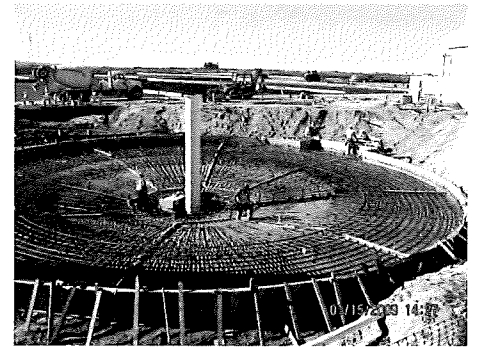
Santa Maria Digester No. 4 Base Slab
