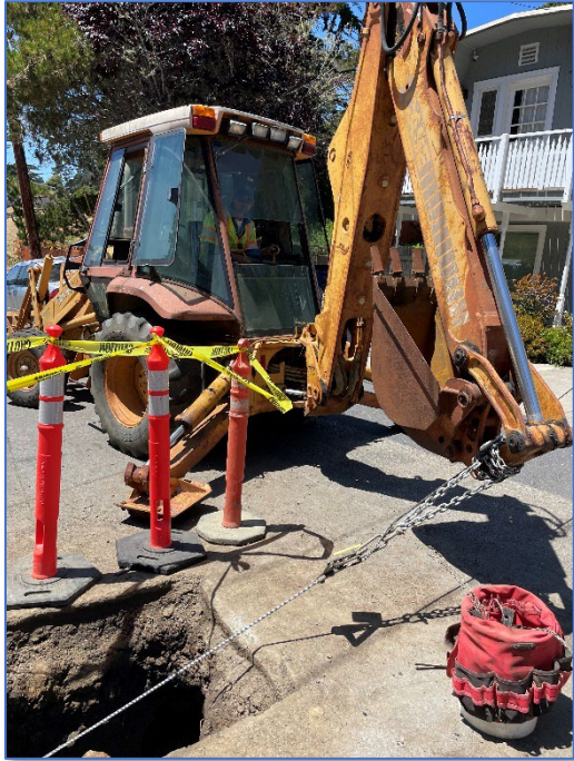
Figure 12: Line pulling on Sheffield Drive
