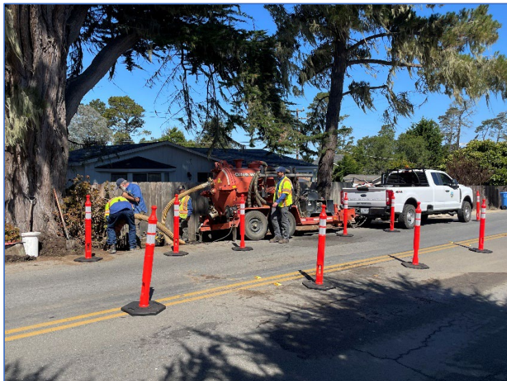
Figure 10: Burton Drive repairs
