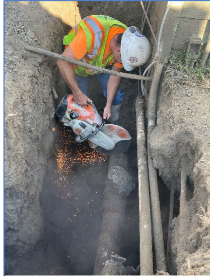
Figure 7: Rodeo Grounds facility plumbing repairs
