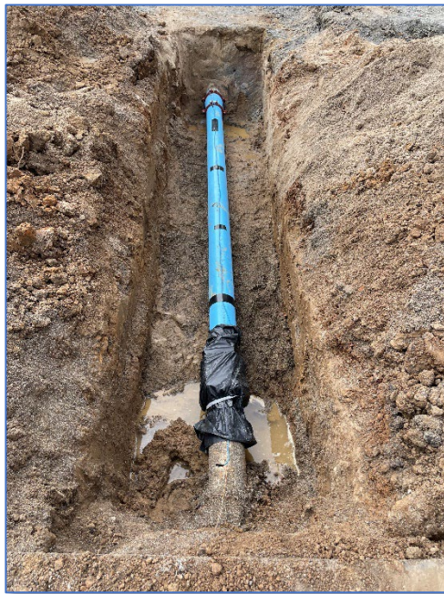
Figure 6: Pineknolls Drive water main repair
