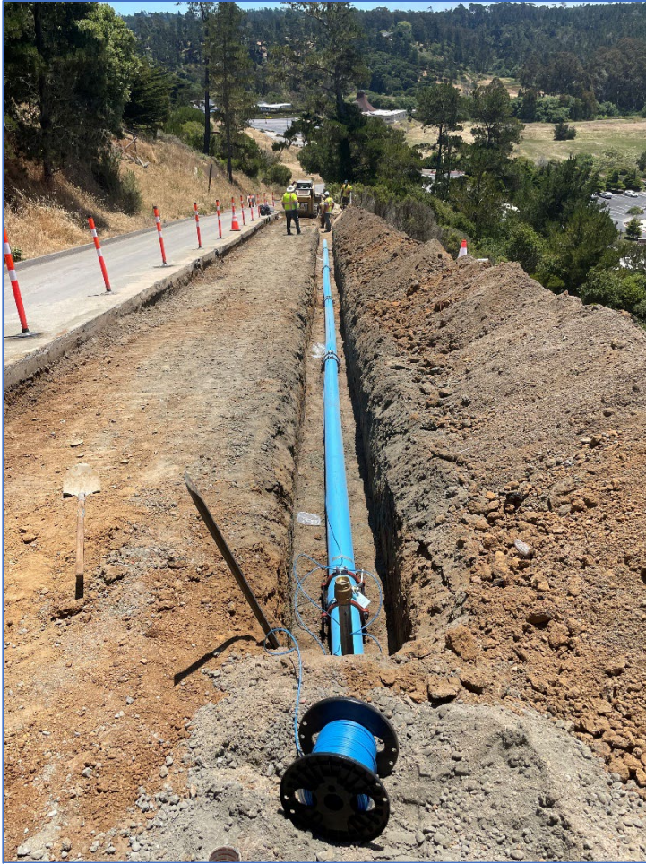
Figure 4: Pineknolls Drive water main replacement
