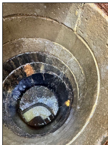
Figure 3: Stormwater infiltration
