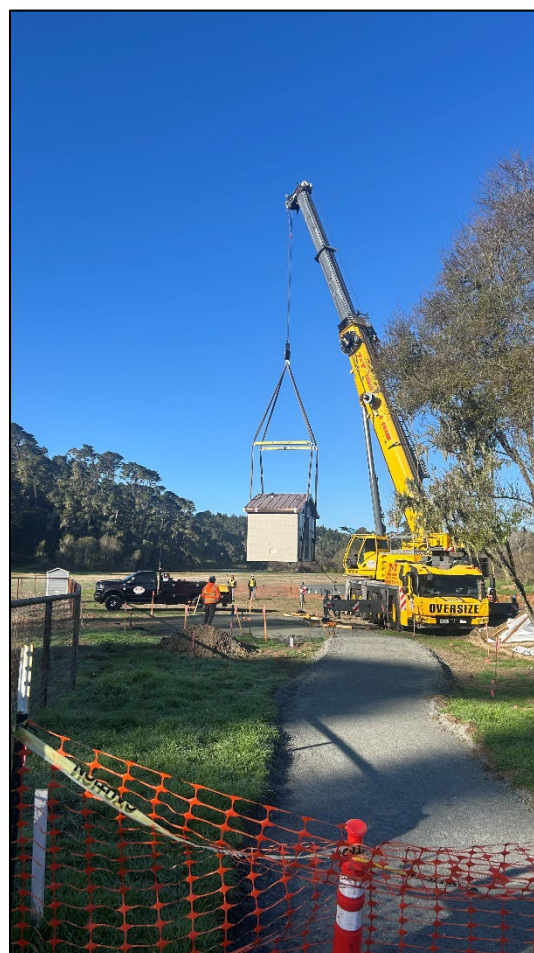
Figure 21: The swing into place
