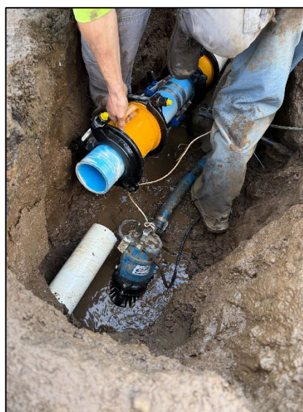
Figure 10: Water Main repair in progress
