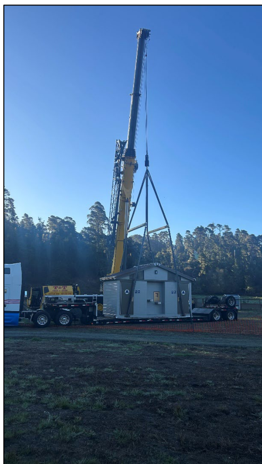
Figure 20: The big lift
