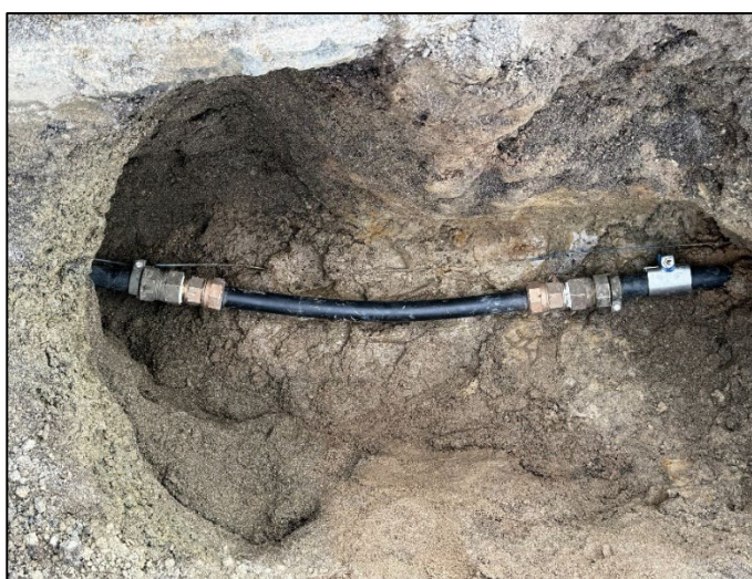
Figure 4: Replacement HDPE service line
