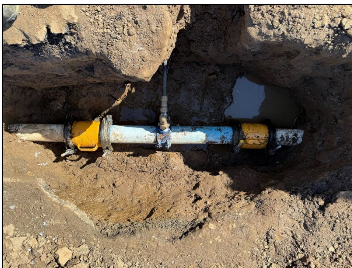
Figure 11: Finished repair before fill
