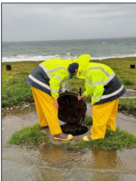
Figure 2: Inspection of manhole for Inflow and Infiltration (I&I)
