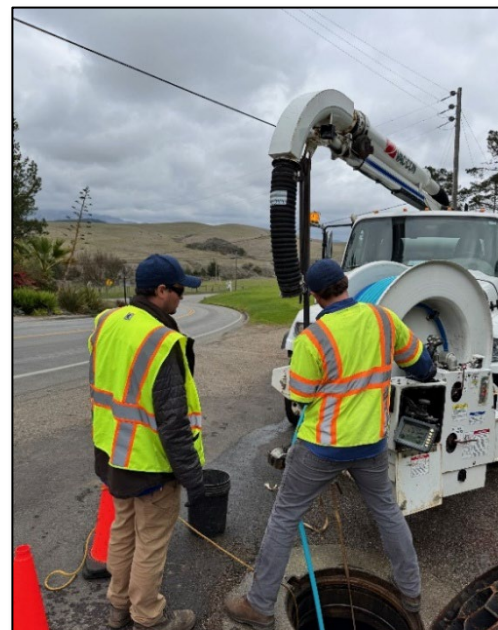
Figure 1: Vac Truck clearing and cleaning
