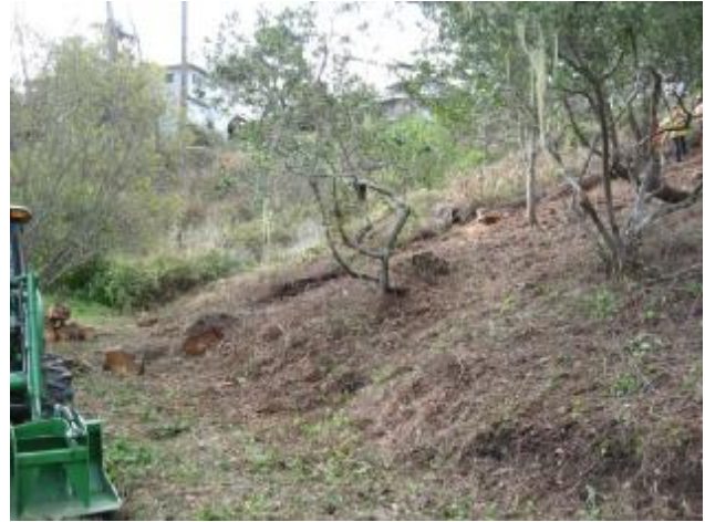
Sta. #2 looking south foreground just cleared
